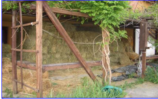
Hay under the deck
